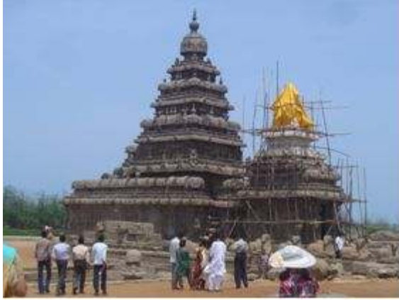
Figure 4: Renovation work at Shore temple by ASI (Source: Author)
