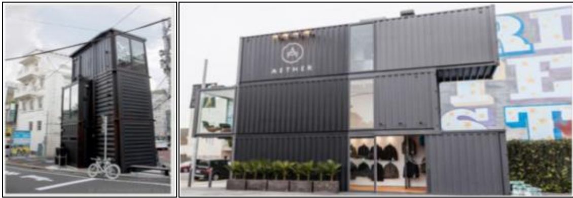
Figure 10 Vertical & Horizontal Placement of Shipping Container
