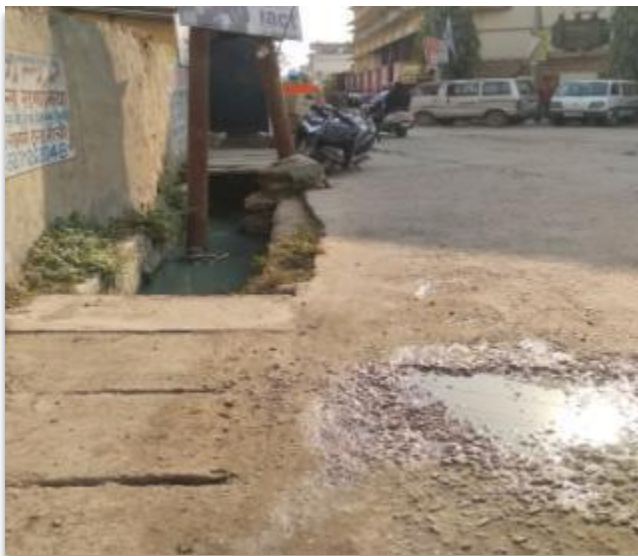
Figure 12: Open sewer, Main road, Ranchi
