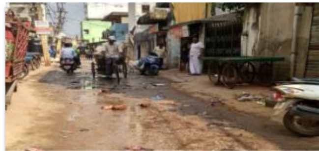
Figure 18: Sewer over flow during rainy season
