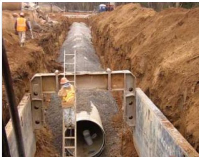
Figure 23: Construction of combined sewer
