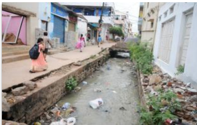
Figure 9: Existing sewer (Open Nallah)
