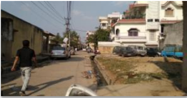
Figure 11: Open sewer line, Hindpiri, Ranchi
