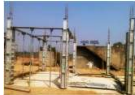
Figure 2. image of special type of form work used for construction made of aluminum.
