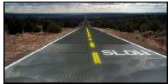
Fig.6:Solar Road with LED Indicators
