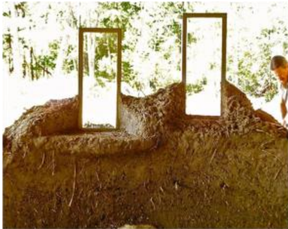
Figure 14: Temporary wooden planks or shuttering can be used to leave space for windows
