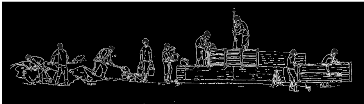
Figure 17: Rammed earth wall construction Source- ( www.madeonearth.com )
