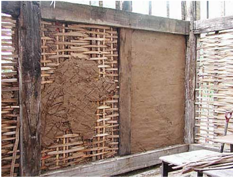
Figure 22: The figure shows portions of wall with exposed wattle weaved into staves and portion of the wall with a daubing
