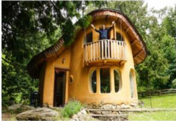
Figure 12: Cob can be used to make buildings upto two stories in height like the cob home we see above.
