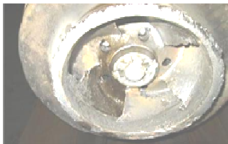
Figure 5.3 Impeller gets completely eroded
